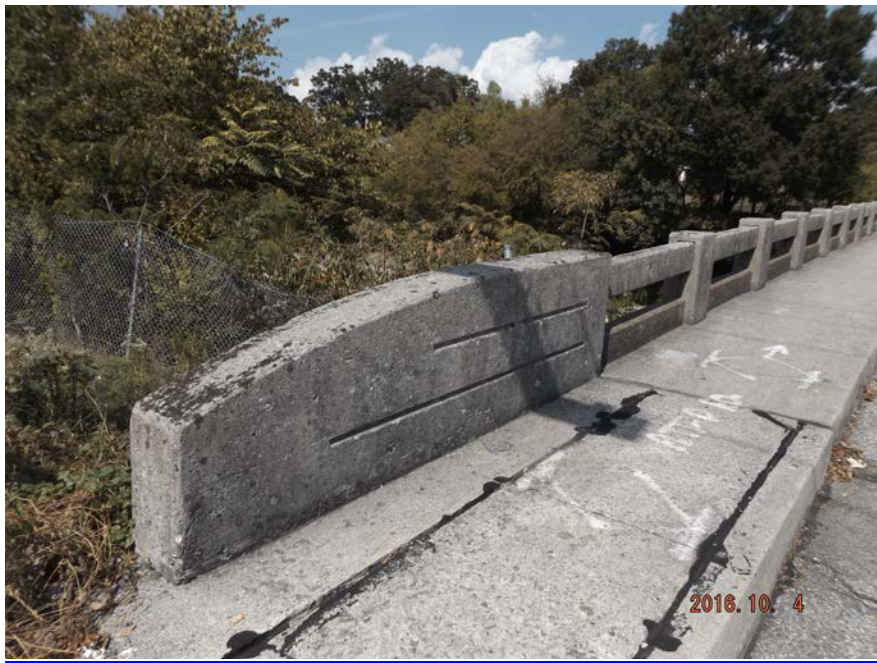
TRAFFIC SAFETY FEATURES - BRIDGE RAIL
