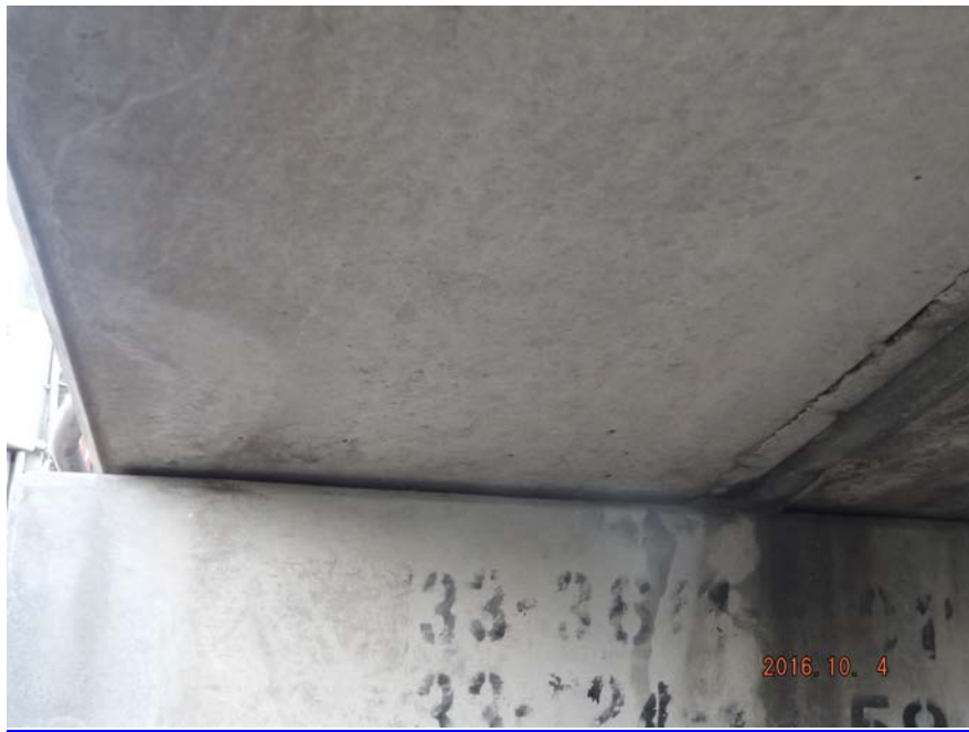
BEARINGS - ABUTMENT - BENT 1
